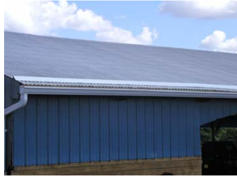
Rain gutters installed on a cattle shed with a snow guard attached to the roof.
