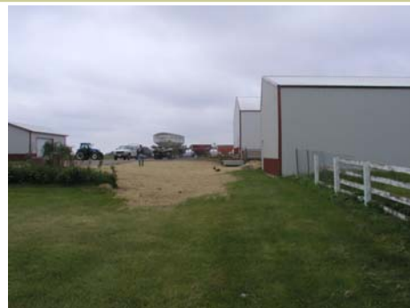
Before (left) and after (right) of a clean water diversion. An old building was removed and channel was shaped to prevent yard water from entering the lot and to carry water from rain gutters on the far machine shed
