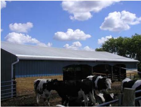
Rain gutters installed on a cattle shed with a snow guard attached to the roof.
